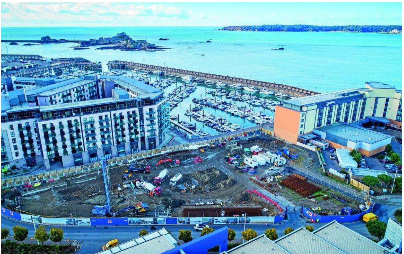
A view of the construction site Picture: Jersey Development Company
